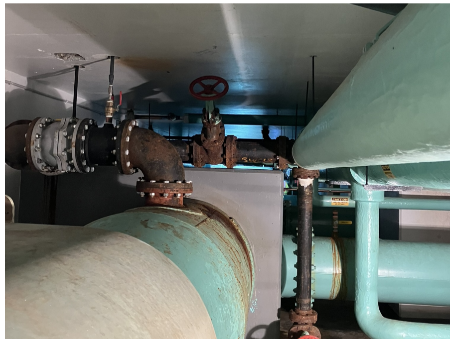
SOUTH EXISTING 250 PIPE TIE-IN TO 1200 PIPE
